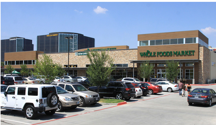
Village on the Parkway SEC Dallas North Tollway & Belt Line Road, Dallas, TX 360,000 SF
